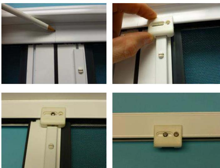
Bring both doors together and mark dead centre, top and bottom. Offer up the shoot bolt keepers as shown and mark for drilling in the centre the large elongated hole. Loosely fix the keepers into place with the screws provided. (This will give you a little adjustment if needed). Check the doors are square and working properly before drilling the smaller hole, and securing the keeper finally into place.
