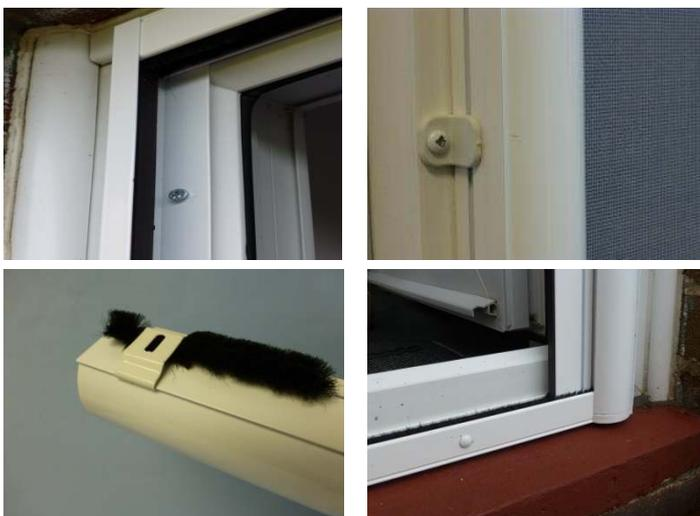
**FACE FITTING** Offer the screen against the frame, ensure the screen is square, then mark the fixing points. Carefully drill the pilot holes. Loosely fit the screen in place using suitable screws. Check operation of screen, before tightening.
