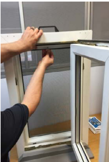
Secure with thumbscrew and lug (bottom outside edge of screen)
