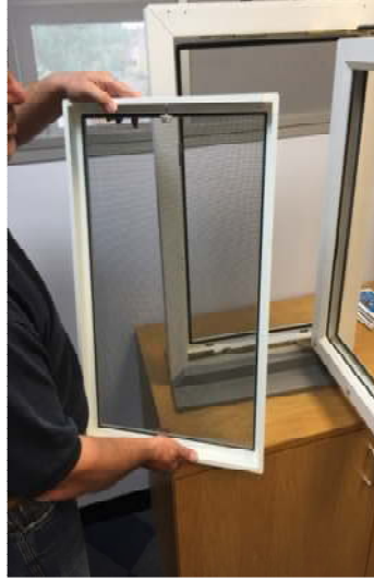
Place screen into aperture
