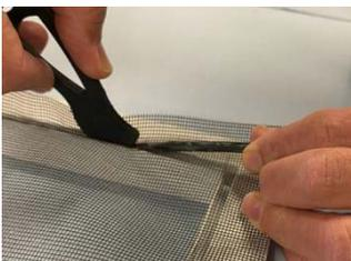
Firstly insert spline at the top and bottom of the frame/mid-bar, and then the sides. Trim spline to length and use the splining tool to push into the corner for a neat finish.
