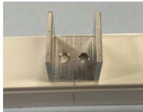
Using the offset midbar profile, slide over the cleat and mark the holes for drilling and screwing.
