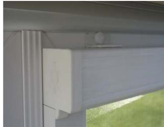
**FACE FITTING** Offer the screen against the frame, ensure the screen is square, then mark the fixing points. Carefully drill the pilot holes. Loosely fit the screen in place using suitable screws. Check operation of screen, before tightening.
