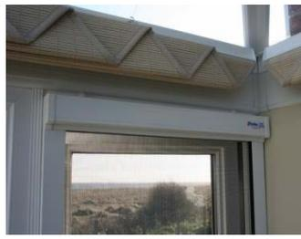
**RECESS FITTING** Offer the screen into the recess, ensure the screen is square, then mark the fixing points for M clips. Remove the screen, Directly fit the M Clips to the top of recess. Click the screen into place. Mark the fixing points for side guides. Directly fix the side guides with suitable screws and fittings if required.
