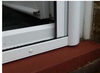
**FACE FITTING** Offer the screen against the frame, ensure the screen is square, then mark the fixing points. Carefully drill the pilot holes. Top guide pilot holes must be 15mm down from the top edge of the profile. The bottom guide pilot holes must be 12mm up from the bottom edge of the guide. Loosely fit the screen in place using suitable screws. Check operation of screen, before tightening.
